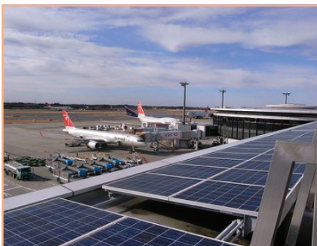
Solar panel installed at Nedumpassery Airport Fig 8.7
