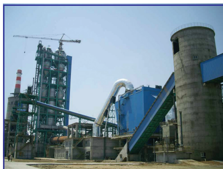
The rotary kiln for the manufacture of cement Figure 8.2
