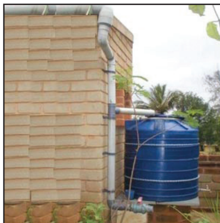
Rain water harvesting - a model
